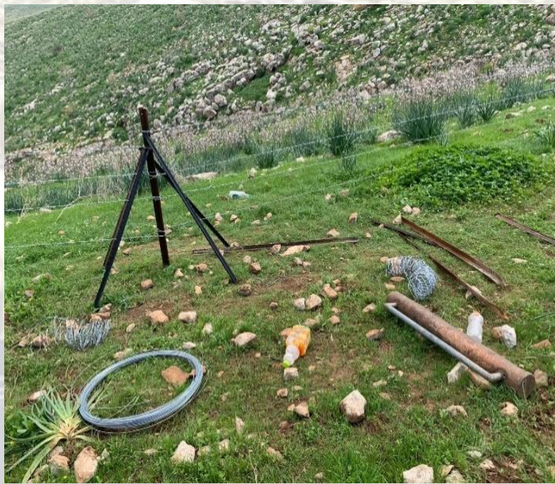
Fence works in Northern Jordan Beqaa Valley
